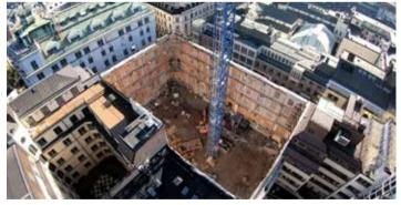
new building that will be constructed will have a higher ceiling height than the previous building. To do this, a new concrete foundation has to be cast an additional 1,5 meter down the ground, below the ground water. The casting process is carried out using the same technique as with the casting of bridge abutments and will be carried out until the summer of 2021. "It is very important that the ground water remains unchanged, otherwise the whole wall can fall."
