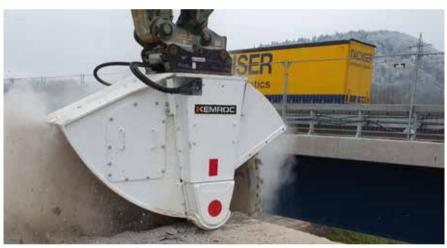
pre-stressed and non-stressed concretes. Using a combination of diamond saw and drum cutter, we made quick progress and achieved a cutting speed of some ten linear meters per hour." He added, "Even with a relatively high wear rate of the tungsten carbide tipped picks, this method proved to be the most economical solution due to high production rates."
