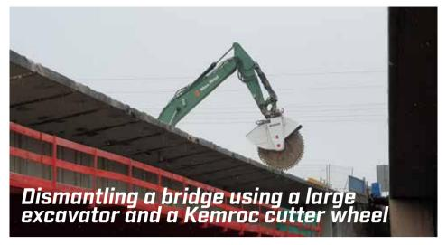
Based in southern Germany, demolition company Max Wild is involved in the demolition of the old Saar Bridge at the Saarlouis autobahn. The plan for demolishing the bridge consisted of breaking it down into sections that could be placed on pontoons and floated to a crushing facility on the riverbank. In order to disconnect the lateral cantilever arms and the concrete slab between the two hollow boxes, the company used one of their 40t excavators with a Kemroc cutter wheel attachment.
