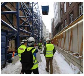
rock. Other stages included sawing of a slot as well as replacement of trusses which had been put up to carry the façade right after the fire.
